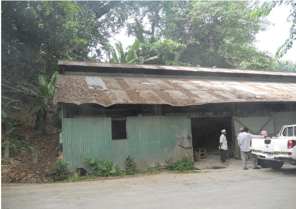
Photo 2; A warehouse in the Kilombero area
